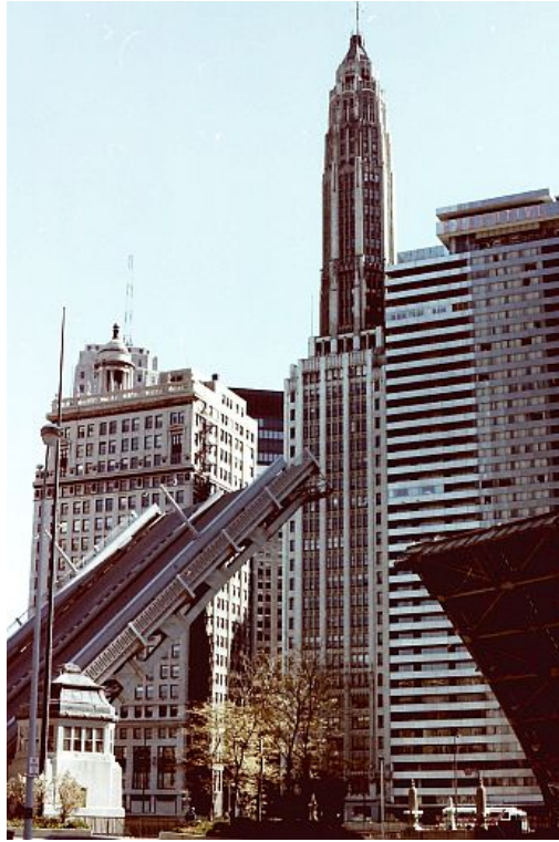
Wabash Avenue Bridge, Illinois 州
